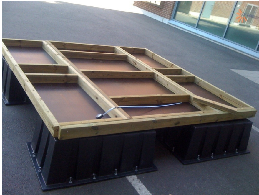
Figure 28 Construction and building up of the ferry
